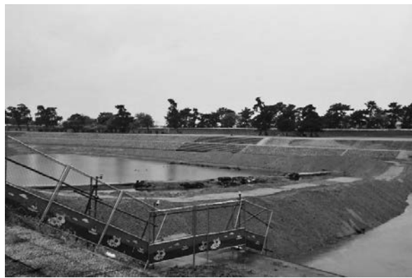
続く河川敷の改修工事
